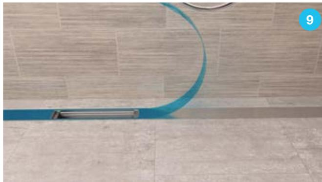
**Step 9.** Remove the stainless steel protector and place the removable grate.
