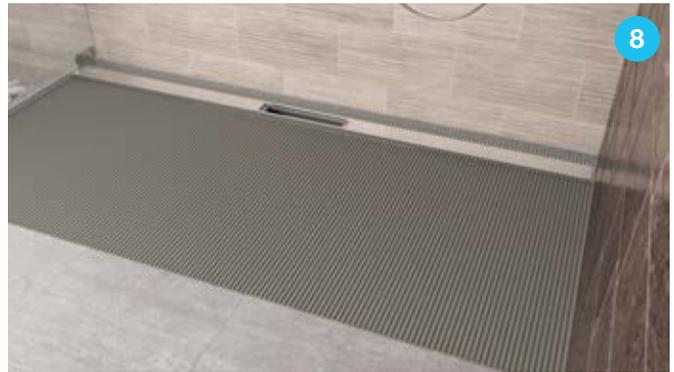
**Step 8.** Apply thin-set and install tile and grout.
