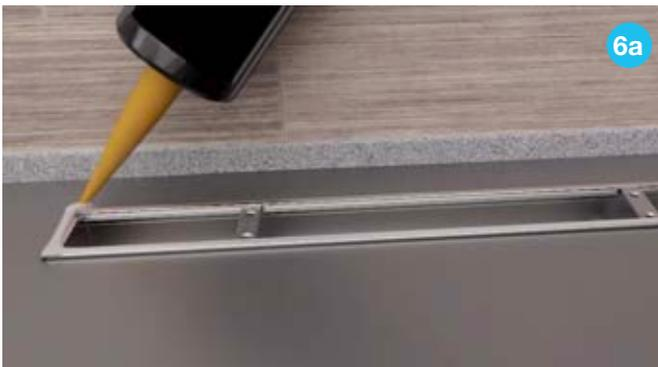
**6a.** Once grate and slider position are verified, apply Sikaflex around the top edge of the base and thin-set to the bottom of the grate.
