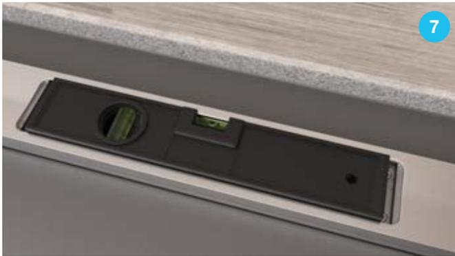
**Step 7.** Verify that the grate is perfectly straight and level before installing the floor. Use enclosed wedges to raise any part of the grate if needed.
