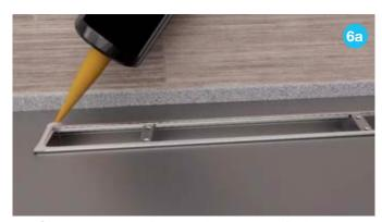
**6a.** Once grate and slider position are verified, apply Sikaflex around the top edge of the base and thin-set to the bottom of the grate.
