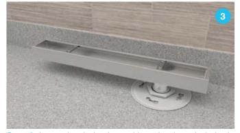
**Step 3.** Insert the drain channel into the threaded nipple. **Step 4.** Trowel mortar to required height.
