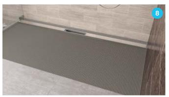
Step 8. Apply thin-set and install tile and grout.
